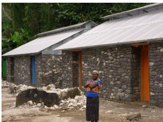
School built with rock cages (gabions) in Bras Gauche – December 2015
